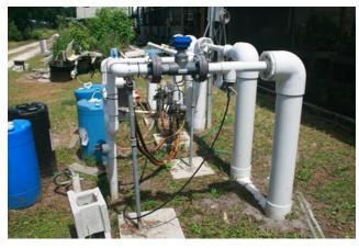
2. The use of strong mineral acids and disinfectants requires a complex injection system to properly meter and control the injection rate, like this system at a commercial orchid nursery.
